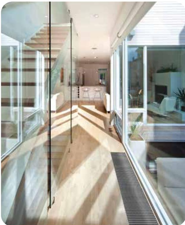
VENTAS forced convection trench heaters with cross flow provide effective solutions as a main heating system as well as being utilized as supplementary heating systems.
